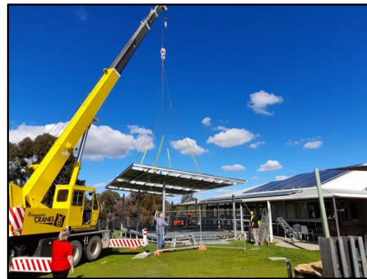
Wangaratta Cranes makes light work of the task.
